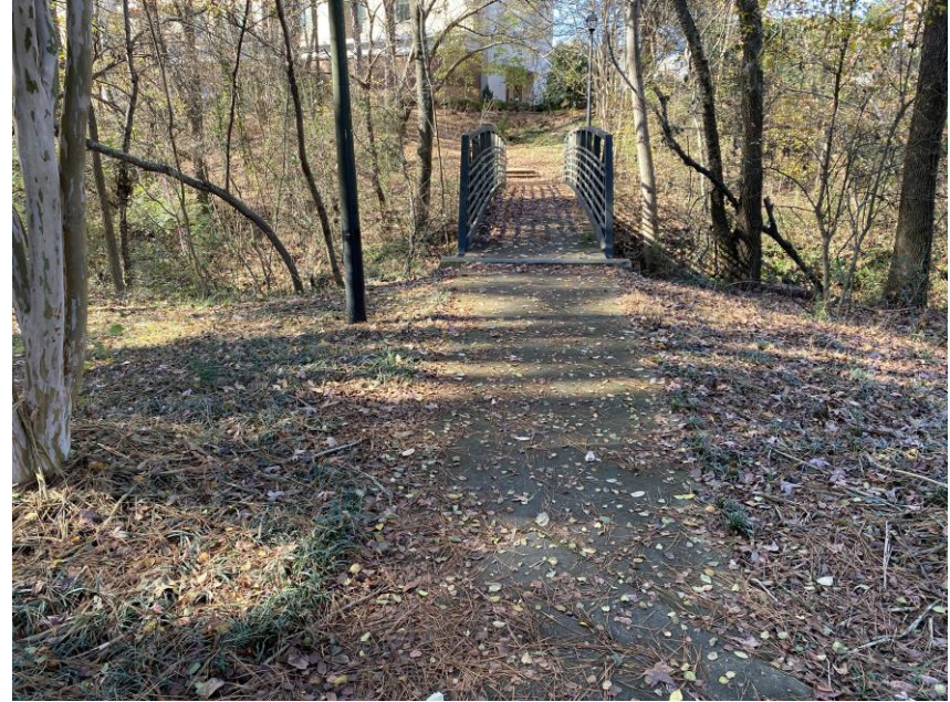
Photograph 8: Existing pedestrian bridge crossing Johns Creek, facing west.
