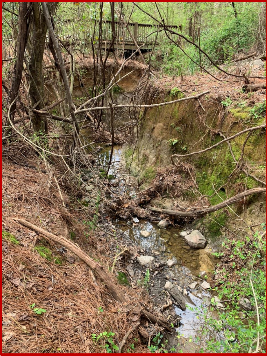
Photo 11: Representative Streambank Erosion
