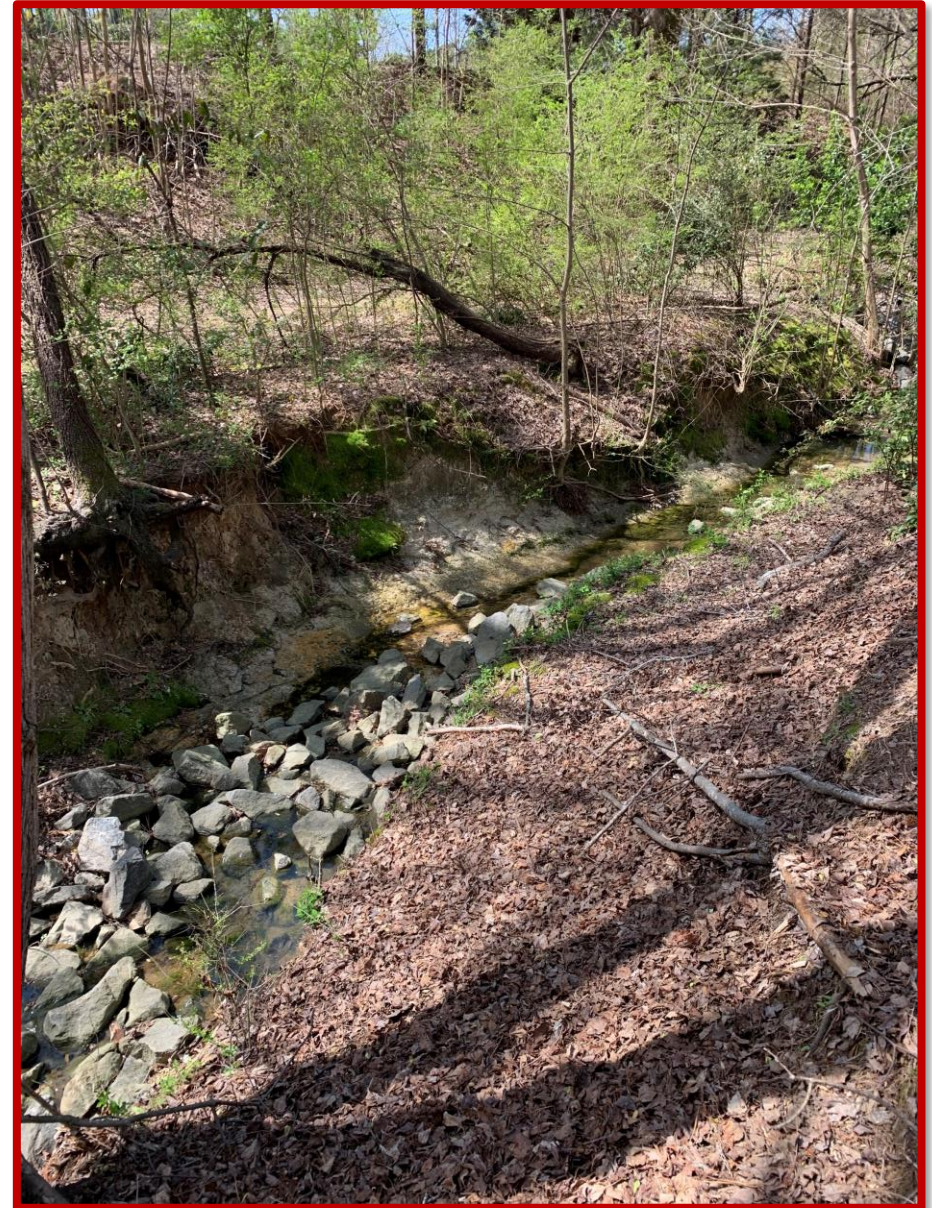
Photo 10: Representative Streambank Erosion
