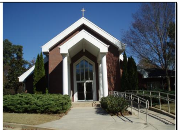
EXISTING MAIN CHURCH ENTRY FROM WEST PARKING LOT
